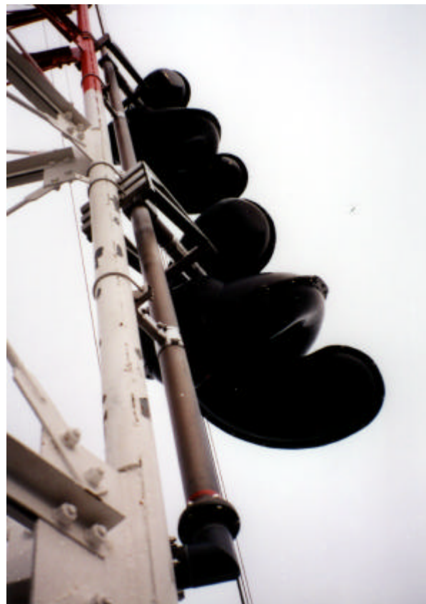
Figure 5 WMGC-FM ERI, type SHPX-2AE Auxiliary Antenna
