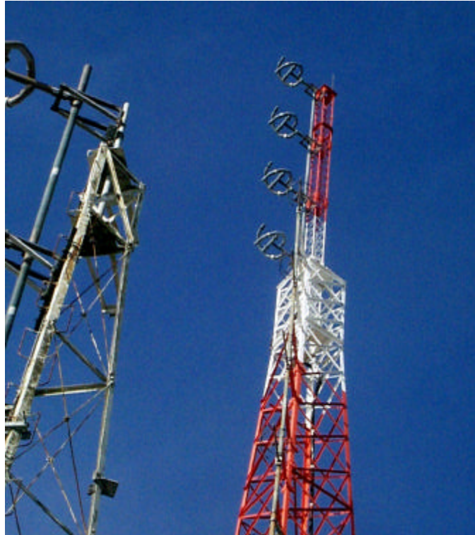
Figure 10 KDFC-FM ERI, type G5CPS-4AE Main Antenna
