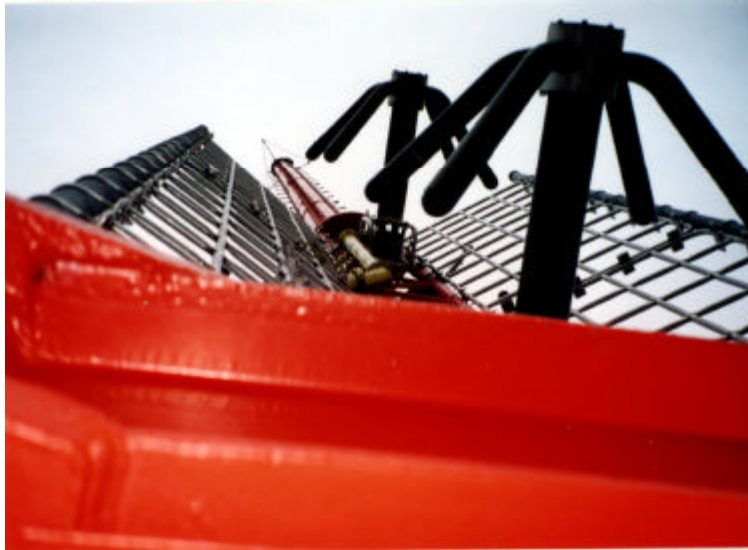
Figure 4 WMGC-FM ERI, type COG-1083-2CA Main Antenna
