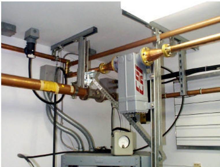
Figure 3 WDHA-FM IBOC Combiner
