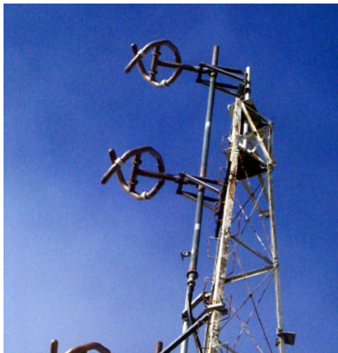
Figure 11 KDFC-FM ERI, type SPHX 2AC Auxiliary Antenna
