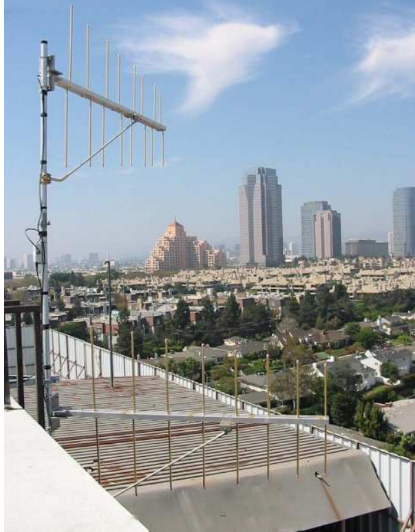
Figure 12 – Transmitting antennas of KCSN booster are vertically polarized log-periodic units oriented to the northwest (upper) and northeast (lower). A power splitter (box mounted on pole) provides equal power and phase to the antennas. Downtown Beverly Hills is visible in the distance.
