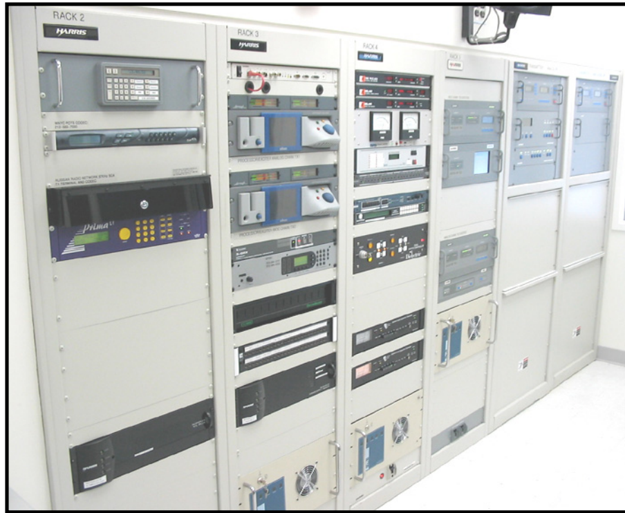
WNYC-FM Transmitter Room. Equipment racks, exciter rack, analog FM transmitter, analog FM/HD radio transmitter. (courtesy WNYC Radio)
