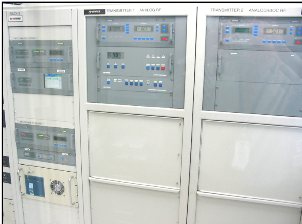
WNYC-FM Transmitter Room. Exciter rack and transmitters. (courtesy WNYC Radio)
